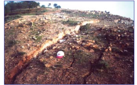
Figure 5: Landslide with cracks in Ait Daoud area
